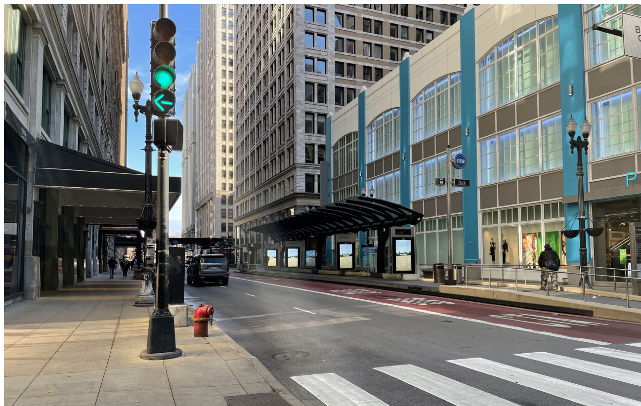
Figure 80: The CTA bus stop at Washington & State combines multiple strategies to minimize bus delay. This stop is located on an island adjacent to a curbside bus lane on the far side of a signalized intersection. A ramp provides access to its raised platform, which allows for near-level boarding.
