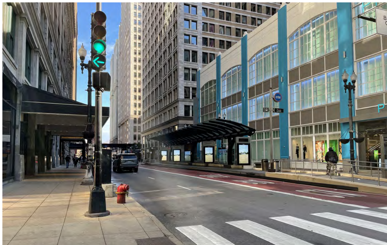
Figure 80: The CTA bus stop at Washington & State combines multiple strategies to minimize bus delay. This stop is located on an island adjacent to a curbside bus lane on the far side of a signalized intersection. A ramp provides access to its raised platform, which allows for near-level boarding.
